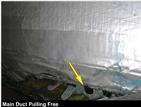
Main Duct Pulling Free
